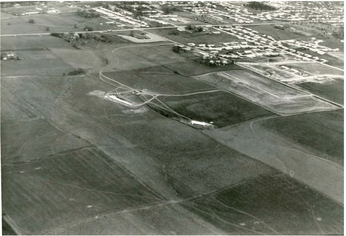
December 1968 - Dorm & Shop Progress
