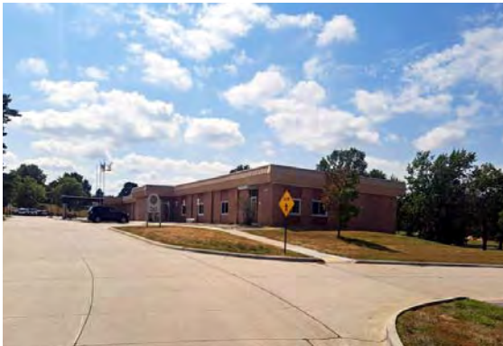
Former Admin. Bldg from where Dorm was. They put a driveway in front of Bldg
