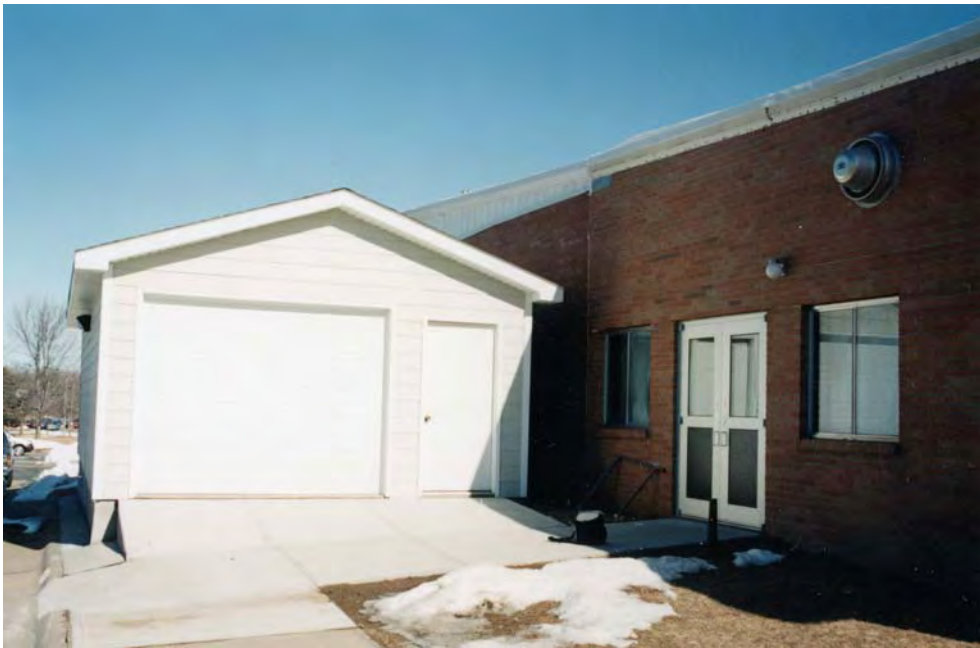
Storage Building built behind Alumni Hall
