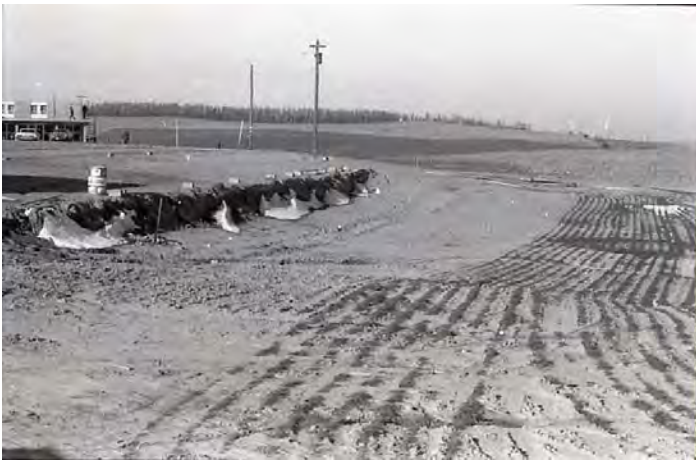
Driveway east of dorm grading
