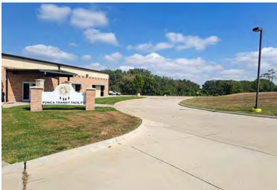
Transit building is where the dorm was with a roadway in front
