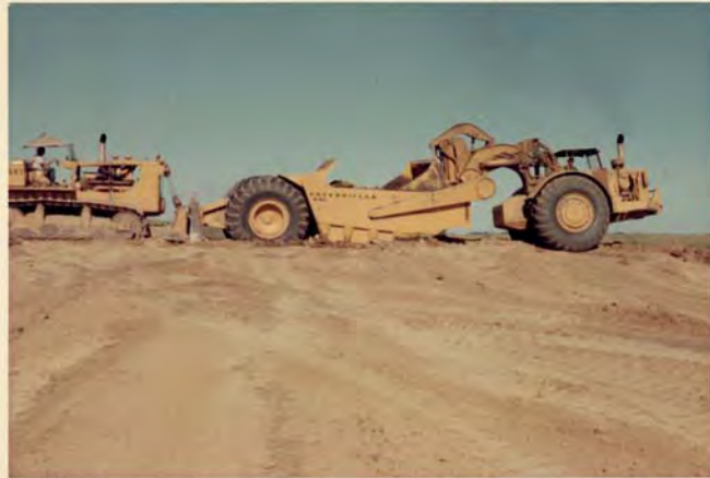
35 yd. earth mover & pusher at N.C.C. 7-25-69.
