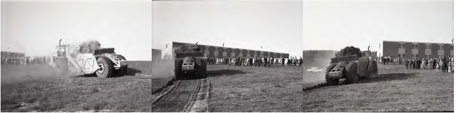
First Dirt Cut
