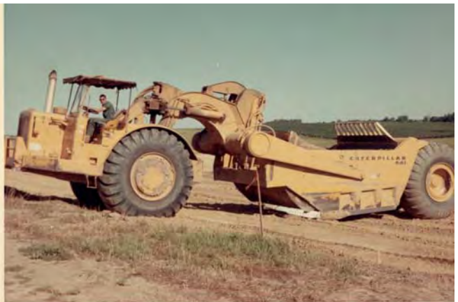
35 yard earth mover at N.C.C. 7-25-69.
