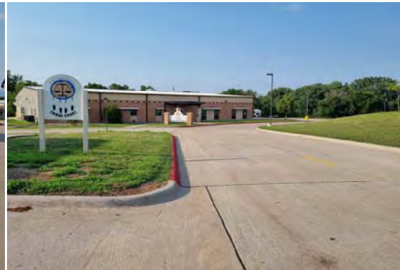
Current building at former Dorm Site
