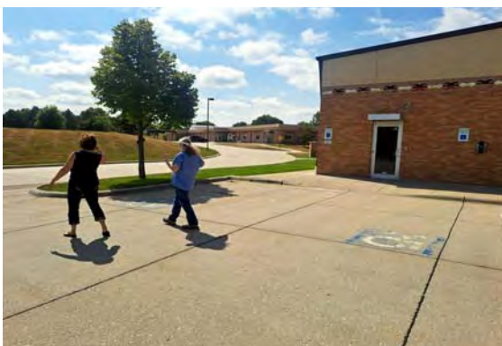
View from east side of Transit Bldg toward Admin Bldg
