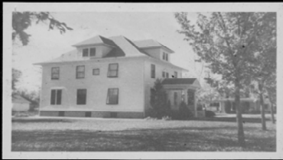
Administration Building (Kodachrome picture)
