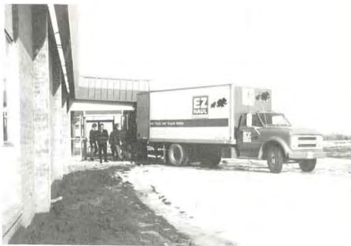
Truckloads of desks, books, and chairs invaded the new building as Mrs. Porter and Sally install shelves in the new library.
