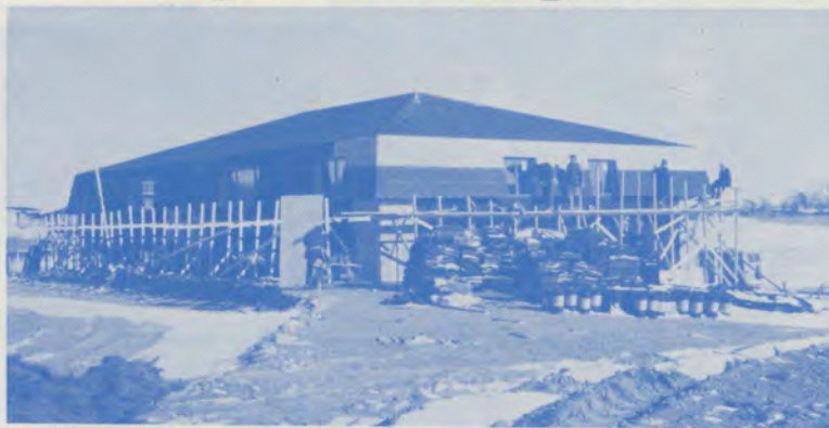
The first week in December the 8-plex appeared as above. It is enclosed and the builders can work through the winter months doing necessary inside work.
