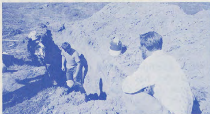
Workmen repairing the break
