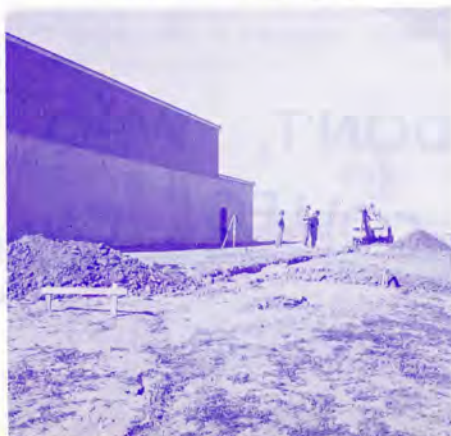
Beginning site preparation
