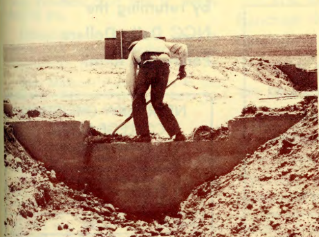
Water Ways for Drainage Control
