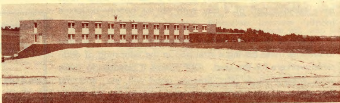
EARTH FILL, SITE READY FOR NEW BUILDING
