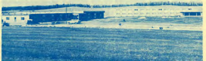
PROGRESS OF CONSTRUCTION
