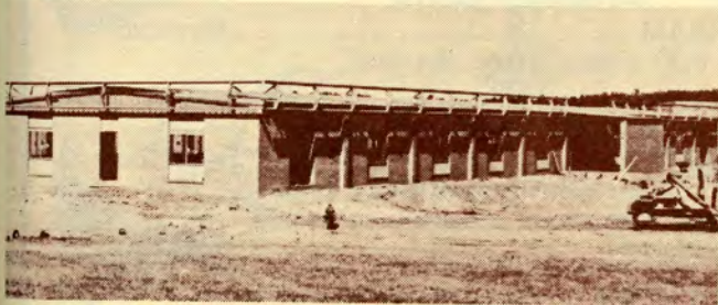
PROGRESS OF CONSTRUCTION
