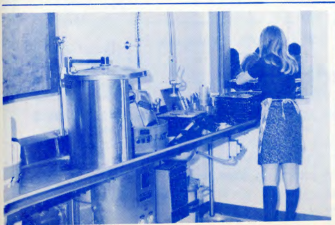
New Kitchen Facilities and Equipment
