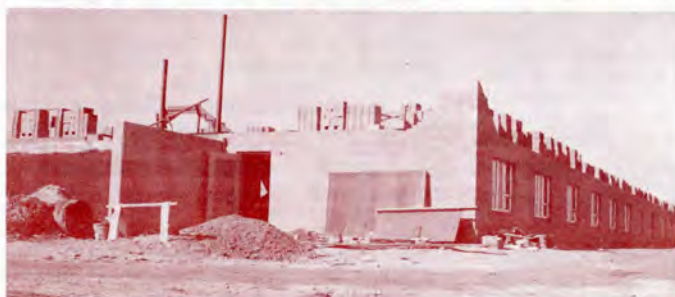
New Dormitory Under Construction
