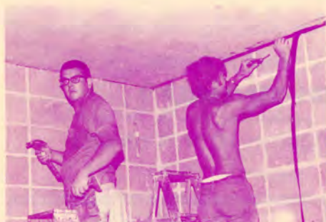
MASKING FOR PLASTERERS
