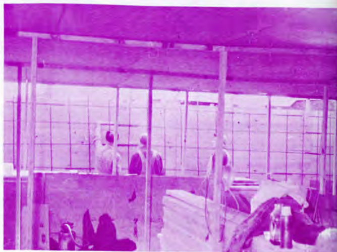
Inside work on the first floor of the Dormitory.
