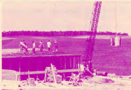
POURING CONCRETE ROOF VIA CRANE
