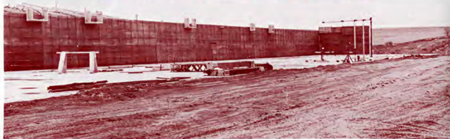
The walls are beginning to rise on the new dormitory. In the background you can see activity on the new workshop building.
