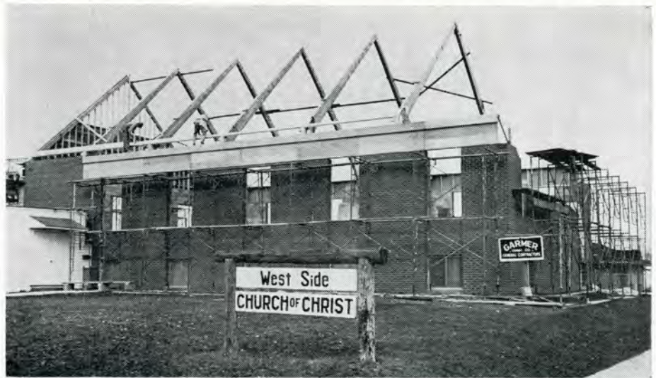
Construction as it appeared the early part of May.
