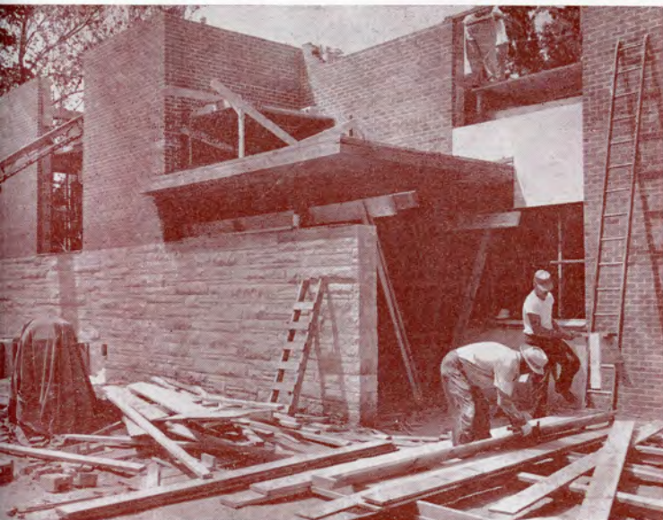
Entrance to New Structure
